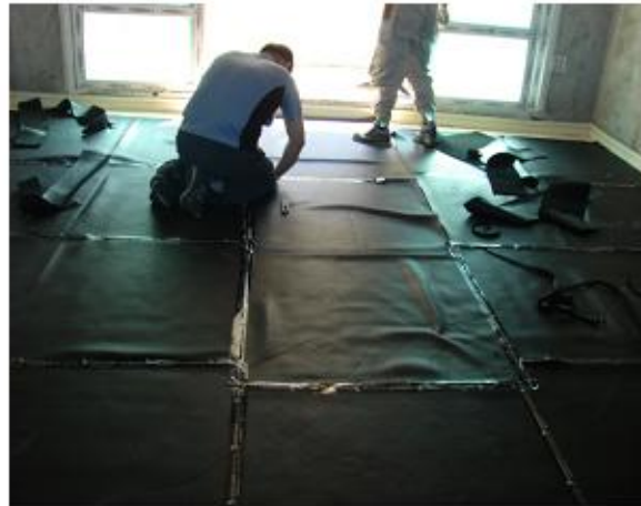
(c) 완충재(EPDM FOAM) 설치
